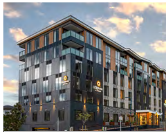
Dec 2020 Completed and Opened
