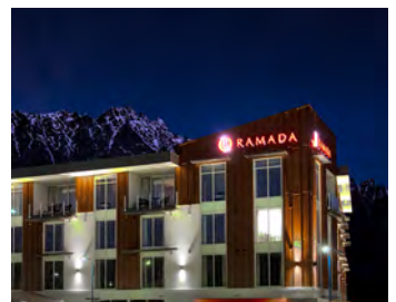
June 2016 Completed and Opened
