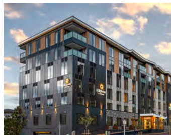
Dec 2020 Completed and Opened
