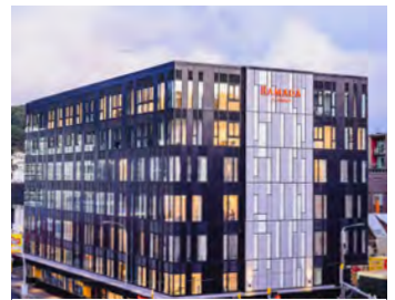
June 2021 Completed and Opened
