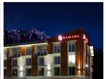
June 2016 Completed and Opened
