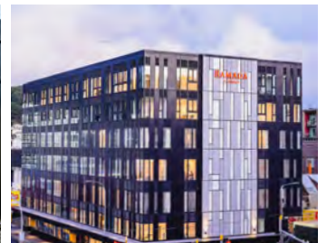
June 2021 Completed and Opened
